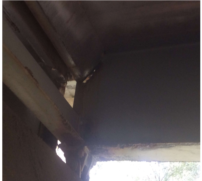
PHOTO 5 Description Span 6 bent 6 girder 1 has small hole in web at haunch with heavy flaking rust and section loss to lower flange at bearing area 2'.
