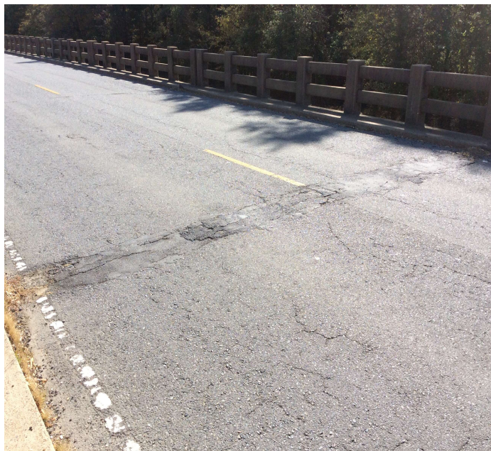
PHOTO 3 Description Wearing surface - Bent 10 (cracking)
