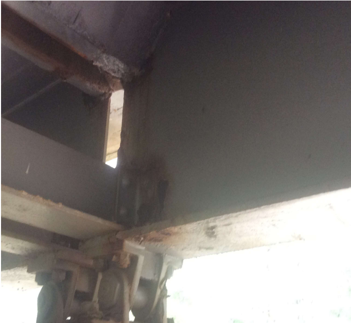
PHOTO 3 Description Span 10 at bent 11 girder 5 has some flaking rust with minor section loss.
