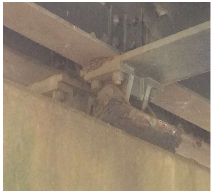
PHOTO 2 Description Bent 14 bearing 2 heavy flaking rust and froze at full tilt.
