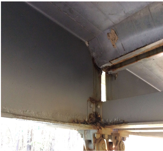
PHOTO 1 Description Span 2 Girder 5 @ Bent 2 (corrosion)
