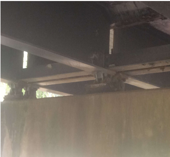
PHOTO 3 Description Bent 14 bearings 1-2 misalignment.
