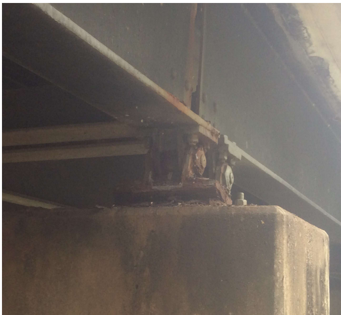
PHOTO 1 Description Bent 14 bearing 5 back has heavy flaking rust with pack rust.
