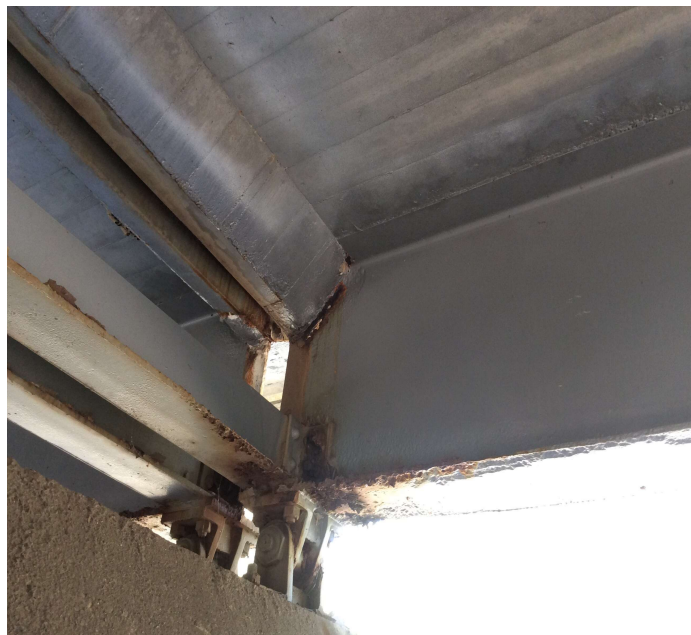
PHOTO 1 Description Span 6 Girder 1 @ Bent 6 (corrosion)
