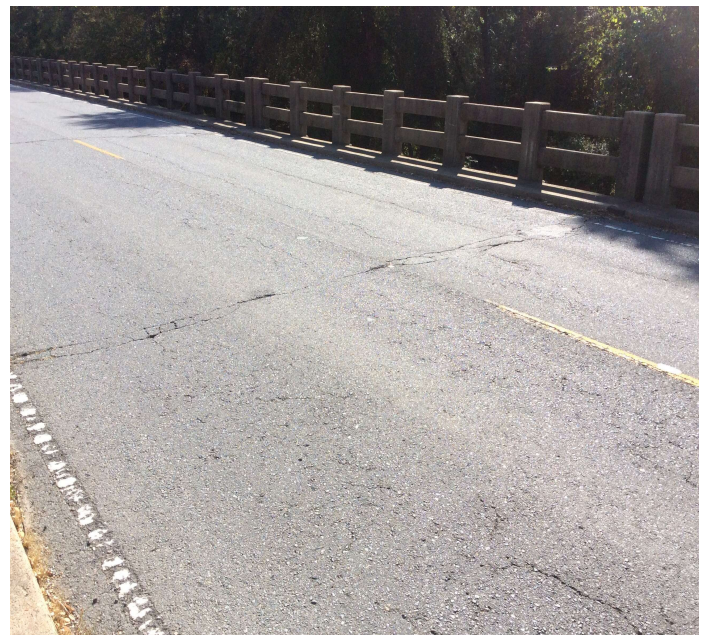
PHOTO 2 Description Wearing surface - Bent 5 (cracking)
