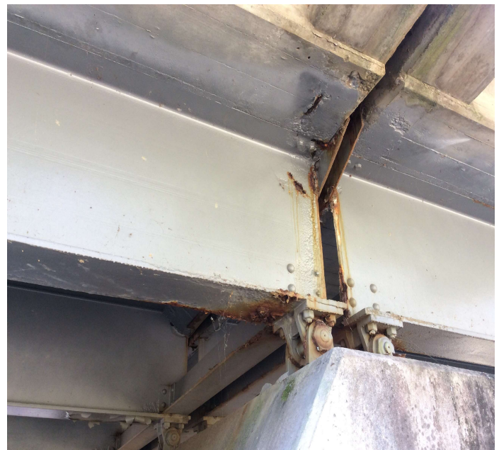
PHOTO 2 Description Span 6 Girder 1 @ Bent 6 (corrosion)
