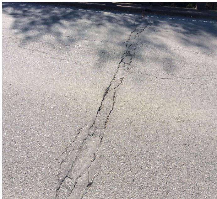
PHOTO 1 Description Wearing surface - Bent 2 (cracking)
