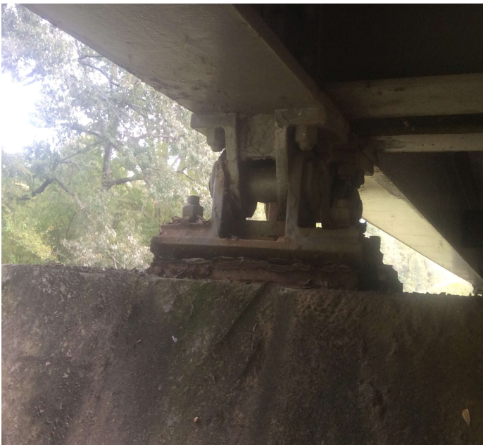
PHOTO 4 Description Bent 11 bearing 1 has heavy corrosion to bottom of bearing and masonry plate. Common all bearing this bent.
