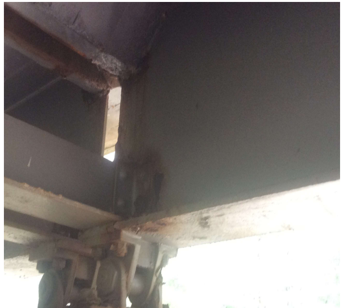
PHOTO 5 Description Span 10 at bent 11 girder 5 has some flaking rust with minor section loss.
