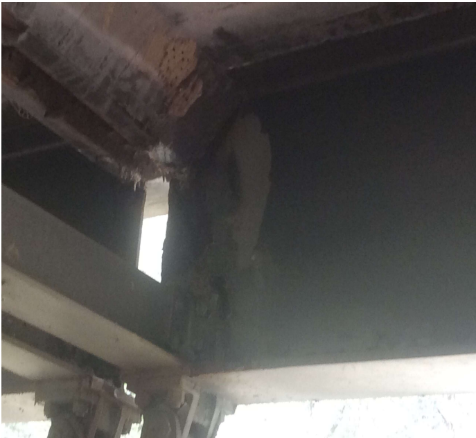
PHOTO 4 Description Span 12 at bent 13 girders 5 has flaking rust to girder end.
