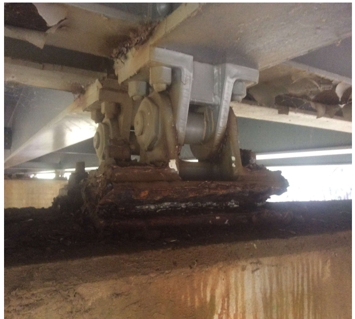
PHOTO 6 Description Bent 12 bearing 3 heavy flaking rust with pack rust.
